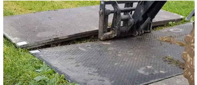
TuffTrak mats are laid out prior to starting a project to help protect the turf from any damage.
